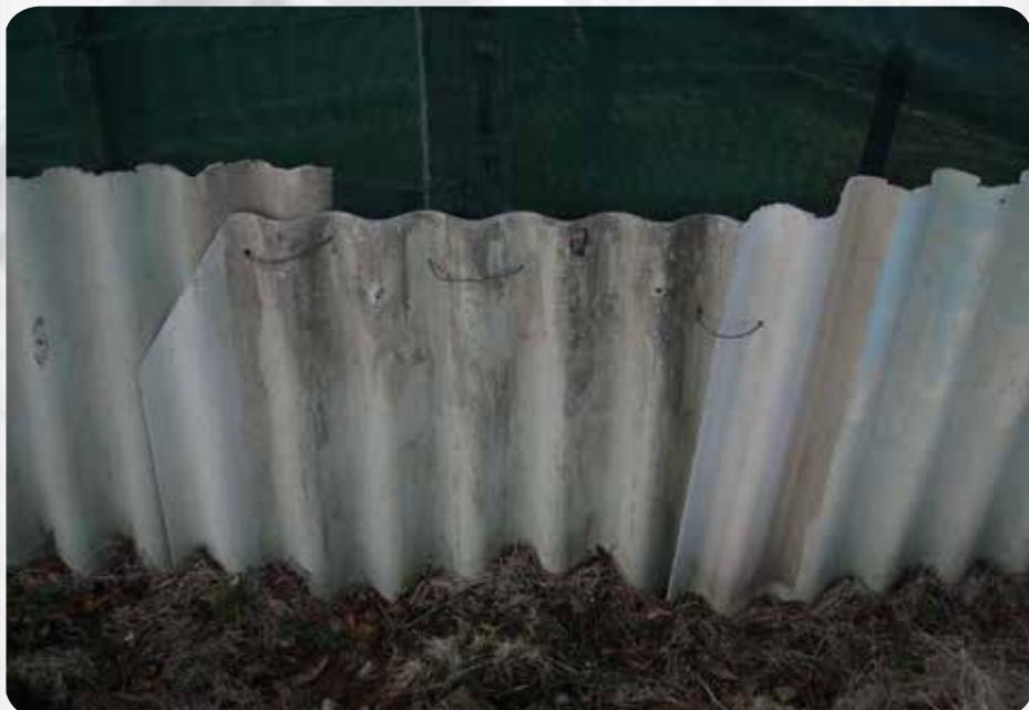
*Super 6 corrugated sheeting - commonly used for roofing, wall cladding and fencing.*
