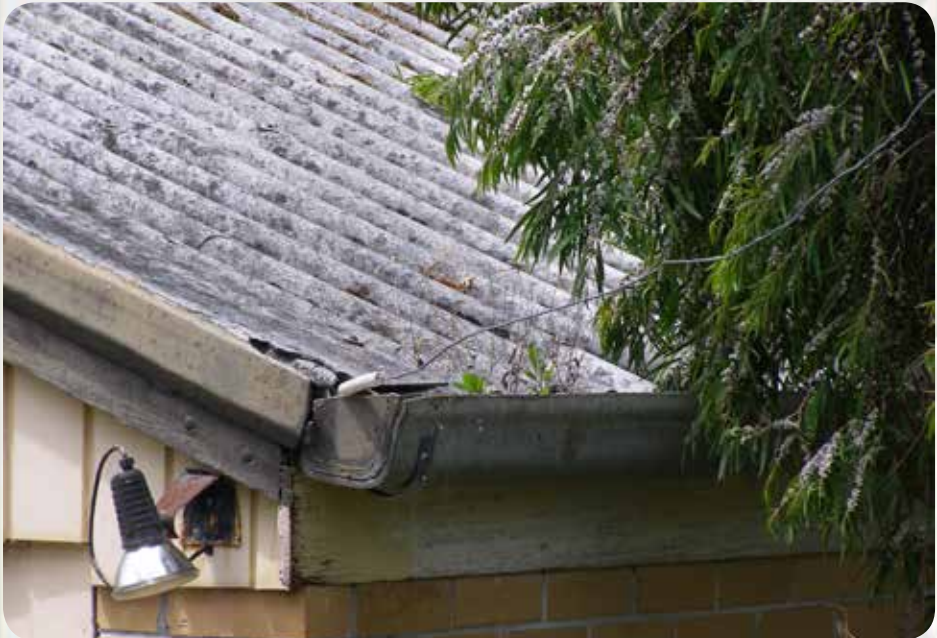
Corrugated roofing, fascia and gutter
