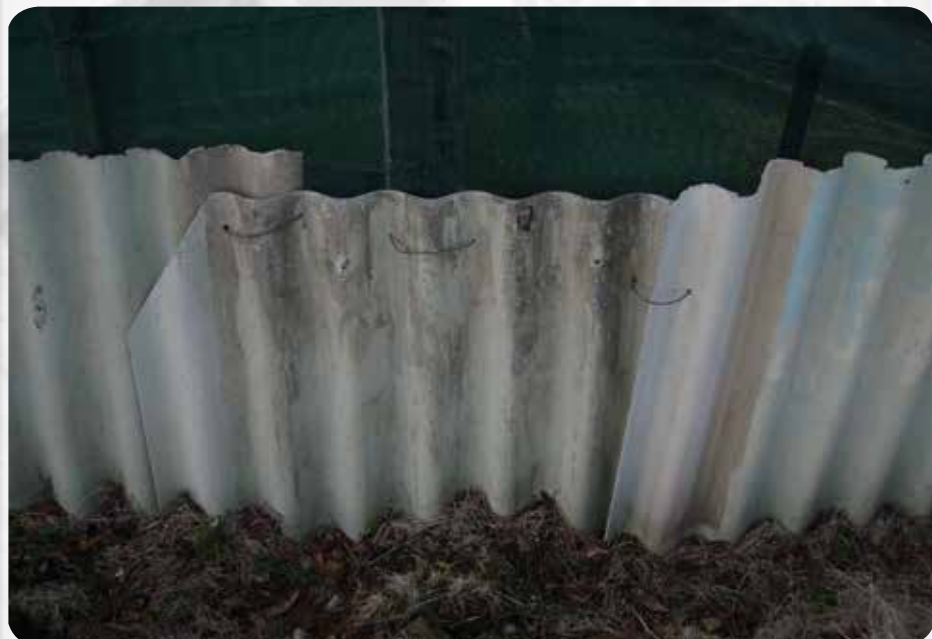
Super 6 corrugated sheeting - commonly used for roofing, wall cladding and fencing.
