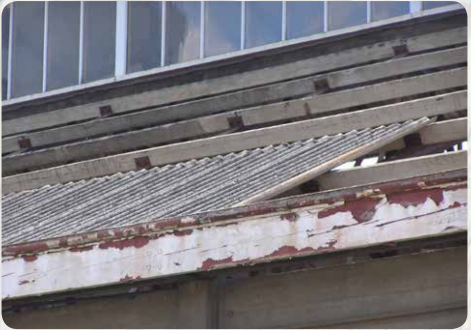
Corrugated roofing panel and fascia / eaves
