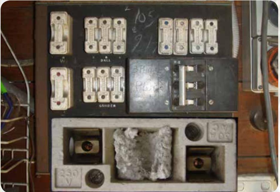
*Fire surround insulating board & heat shields in fuses*
