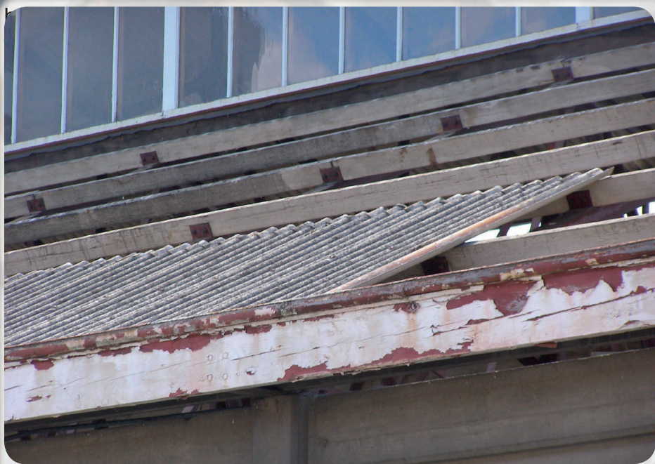
Corrugated roofing panel and fascia / eaves
