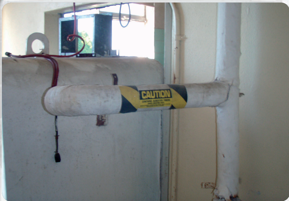
Lagging – for pipes or boilers
