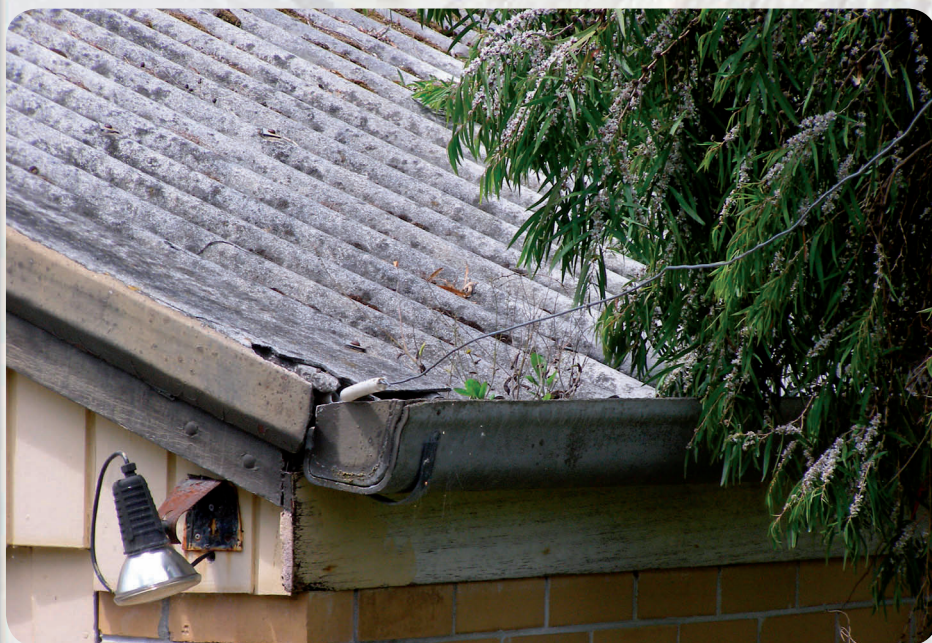
Corrugated roofing, fascia and gutter
